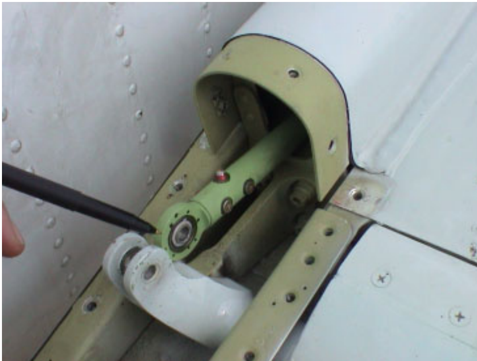
Figure 10. Photograph of the test airplane's right elevator control tab pushrod contacting the crank fitting.
