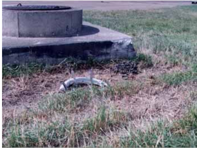
Fig. 1-26 Abrasion Marks and Rubber Deposits
