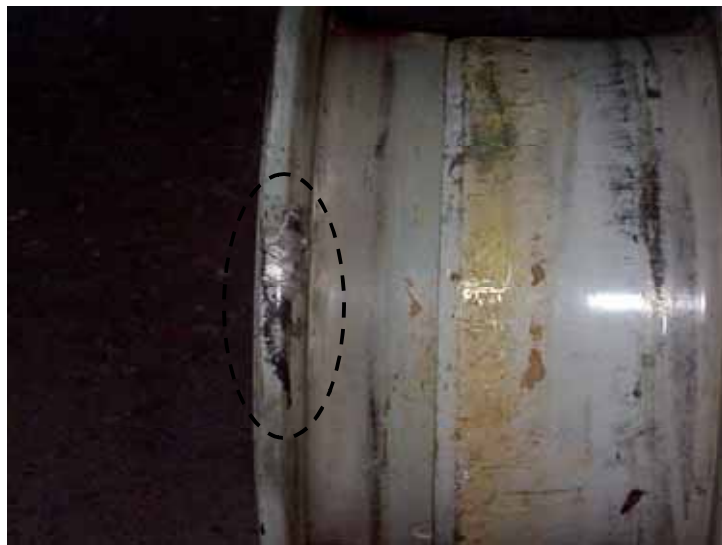
Fig. 1-9 Left Flange Dented and Deformed (circled area)
