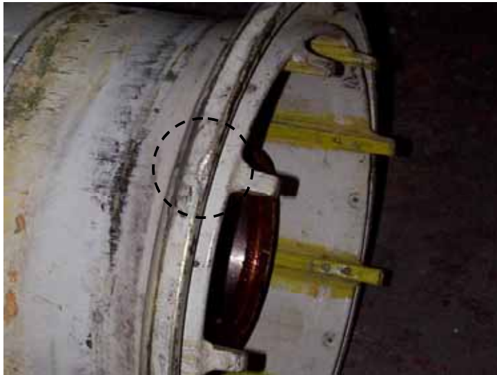
Fig. 1-10 Right Flange Dented and Deformed (circled area)
