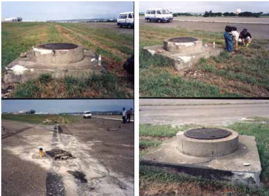
Fig. 1-30 Manhole Struck by Nose Gear
