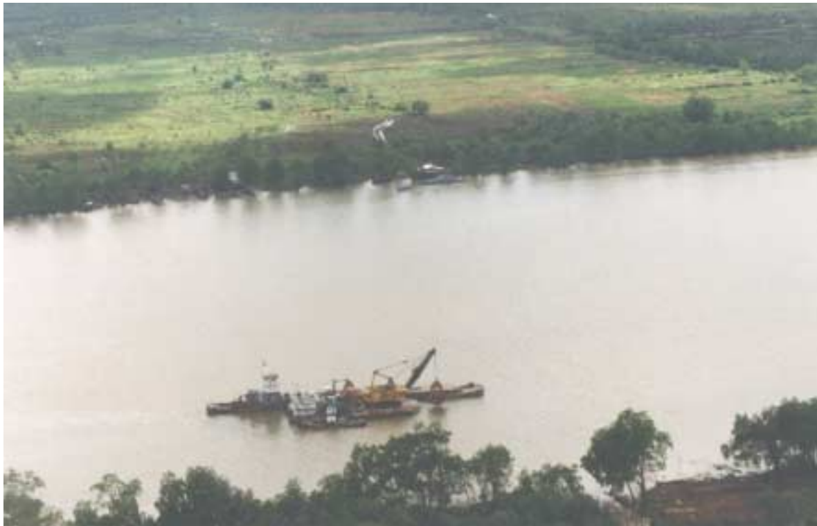
Figure 6.b Debris recovery using dredge
