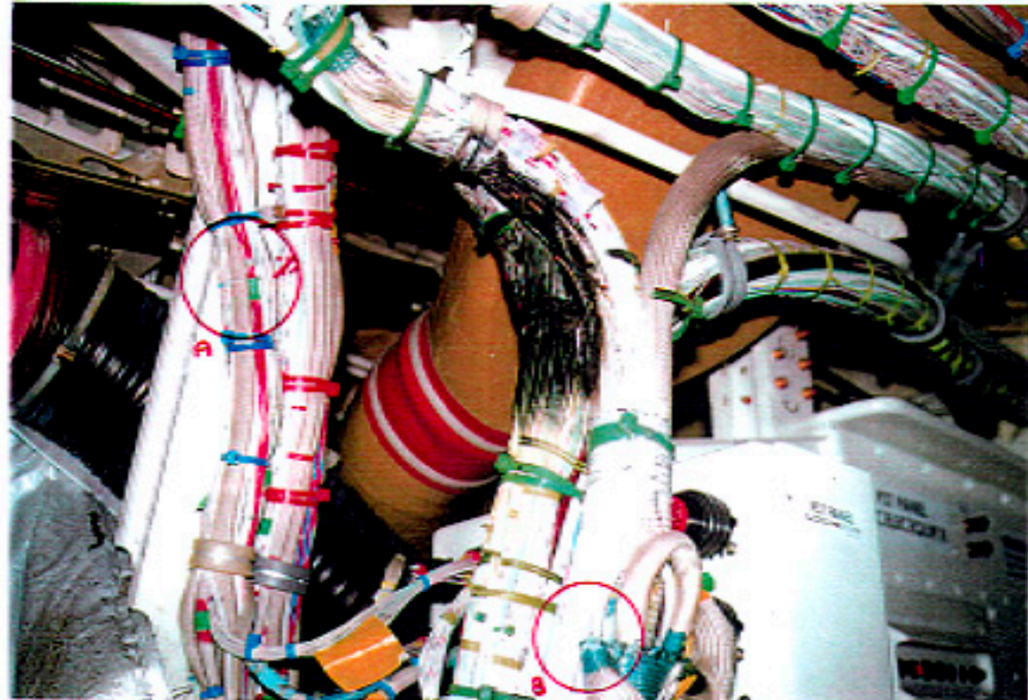
General view of damaged wires after chiller removal, with partially failed loom nearest the camera. Areas identified A and B exhibit wire damage not directly related to the loom failure (see Figure B-3). Of significance, damage at A is approximately at the same height as the failed section of loom.
