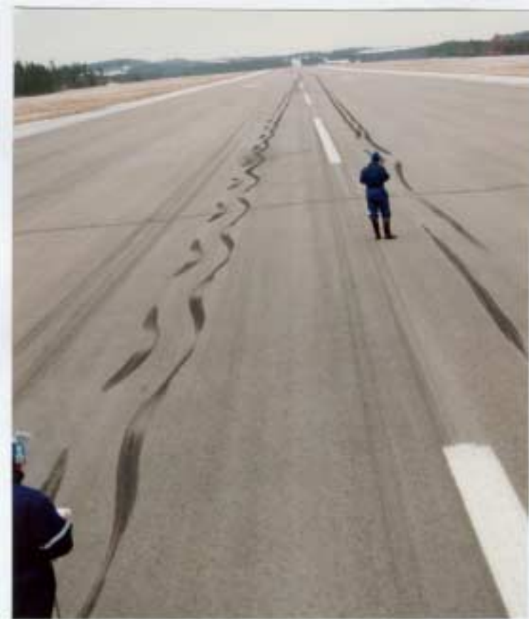
Figure 5. Both main landing gear marks seen to the landing direction. The marks of the left main gear shimmy started at 190 m and the right main gear at 260 m from the touchdown.
