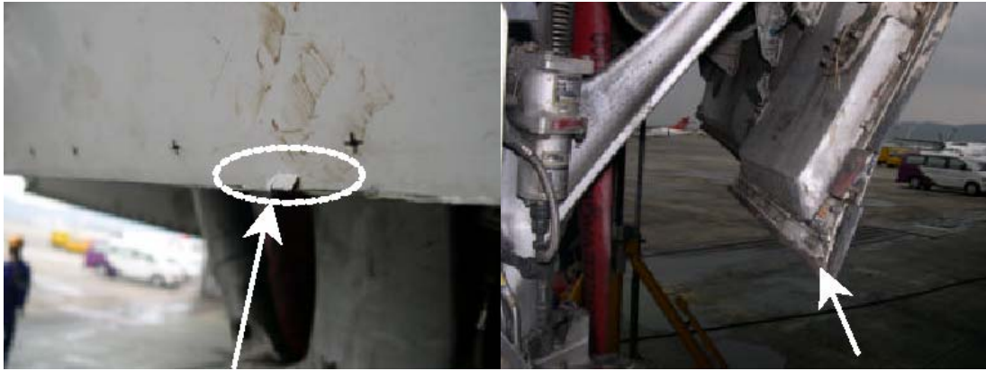
Figure 1.12-4 Deformation and dent to NLG Aft doors
