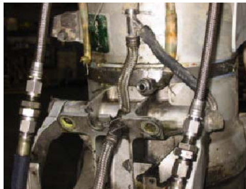
Figure 1.12-5 LH MLG electrical and hydraulic systems damage
