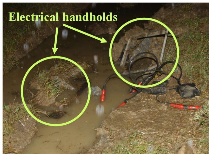
Figure 1.4-2 Damaged electrical handholds
