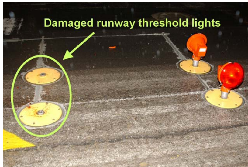
Figure 1.4-1 Damaged runway threshold lights
