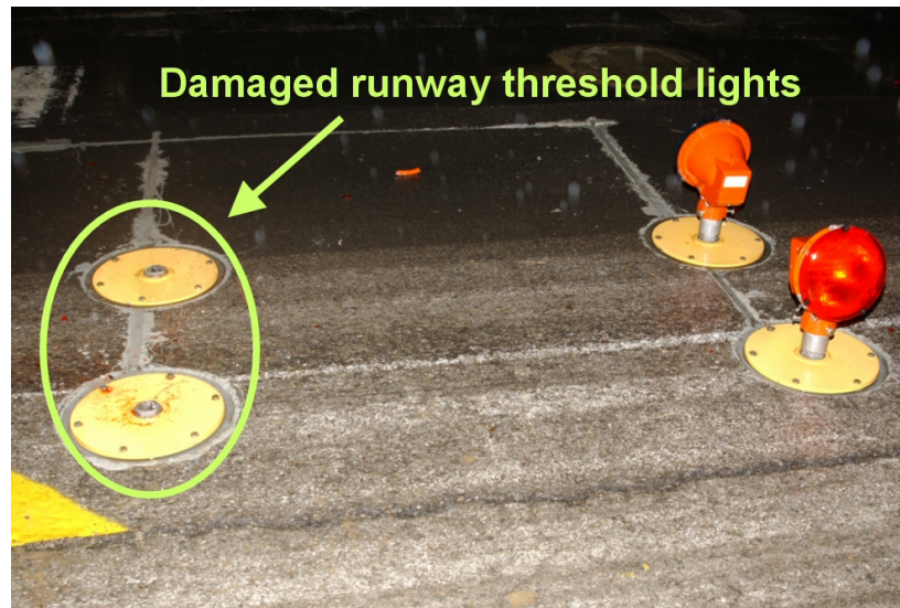
Figure 1.4-1 Damaged runway threshold lights
