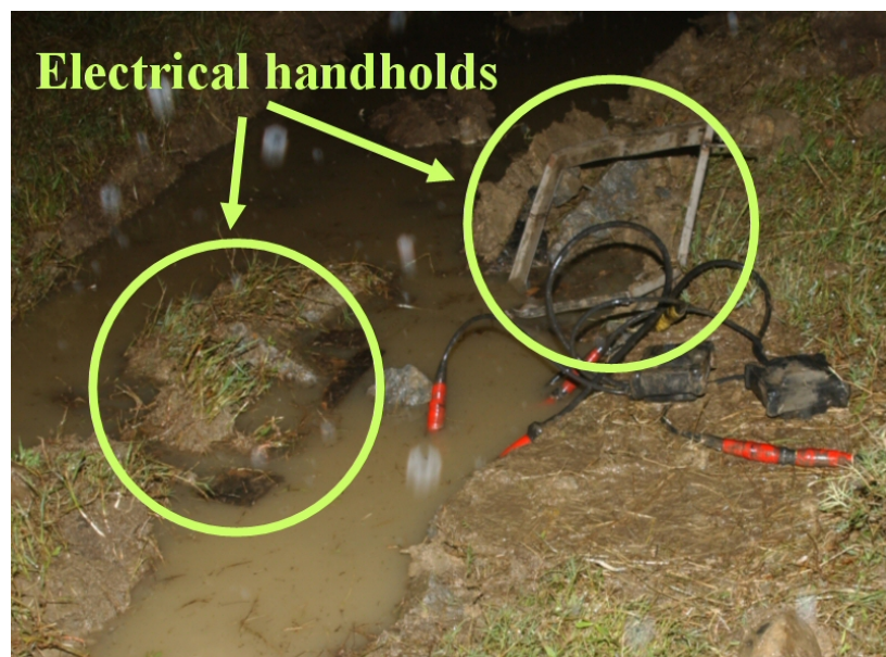
Figure 1.4-2 Damaged electrical handholds
