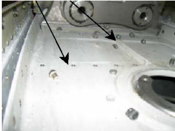
Figure 1.12-17 Upper Panel Pulled fasteners
