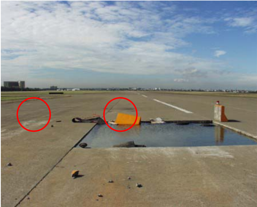
Figure 1.12-3 Initial impact point (shown circled)
