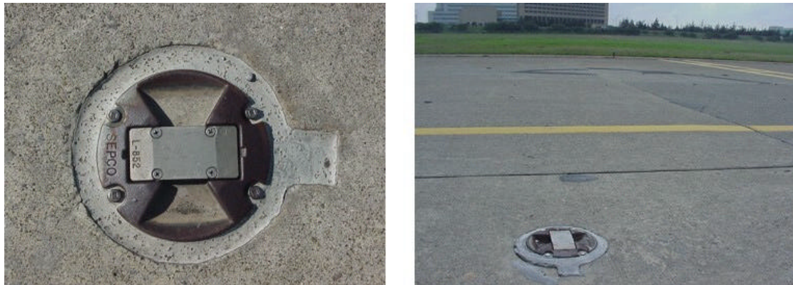
Figure 10-16 Taxiway centerline light installed a curved taxiway section with straight bi-directional light windows (picture taken during site survey)
