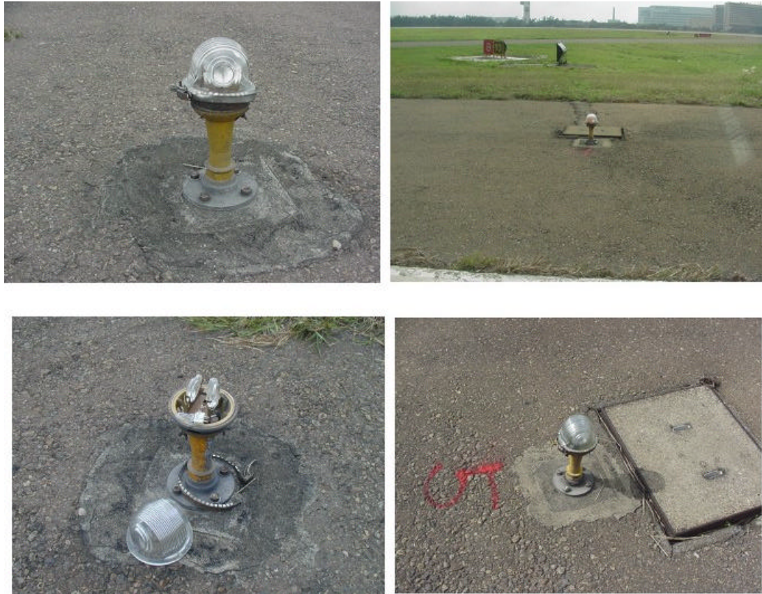
Figure 10-9 Runway 05L/23R and Runway 05R/23L (bottom right) edge lights
