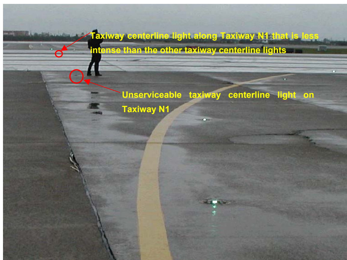
Figure 1.10-10 Status of Taxiway N1 centerline lights close to the threshold of Runway 05R (picture taken on November 4, 2000)
