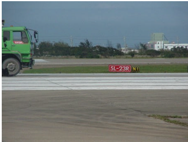
Figure 10-23 Mandatory runway designation sign found only at the right side of Taxiway N1 leading to Runway 05L/23R
