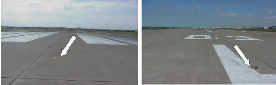
Figure 10-12 05Runway Center Line Light
