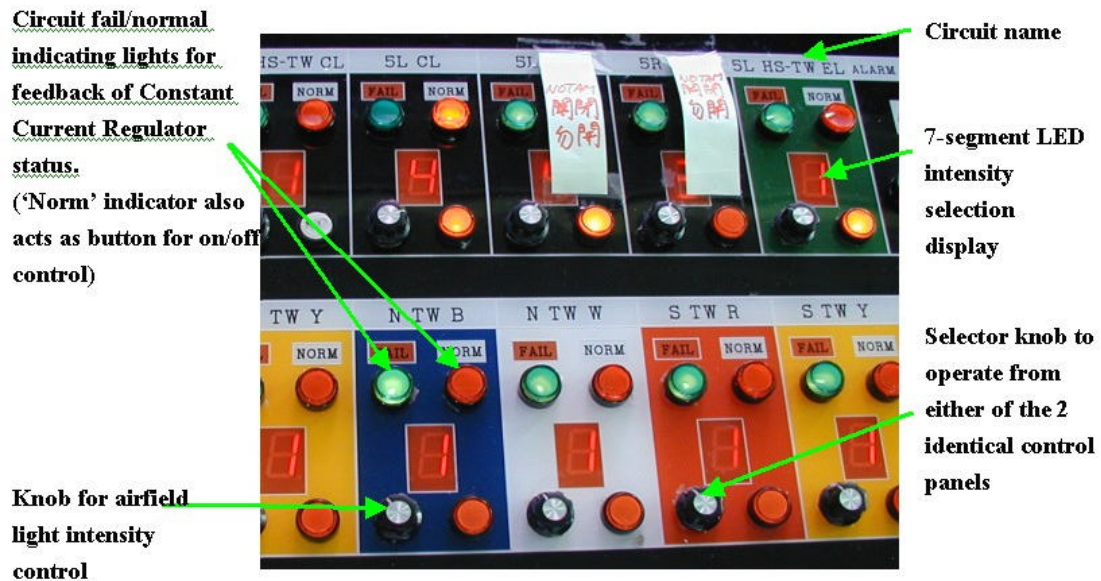
Figure 10-18 Section of airfield lighting control panel (picture taken during site survey) (One of 2 identical panels located in CKS Airport Control Tower)
