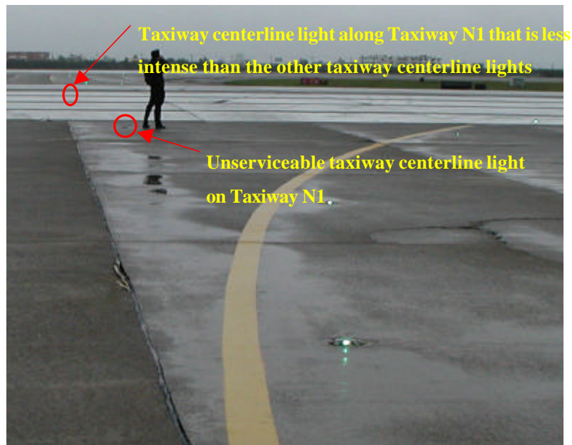
Figure 10-15 Configuration of taxiway center line lights Installed around Taxiway N1 (picture taken during site survey)
