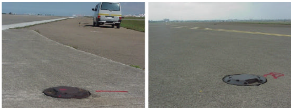
Figure 10-10 Incorrectly oriented inset runway edge lights (L-852) for Runway 05L/23R (left) and 05R/23L (right)
