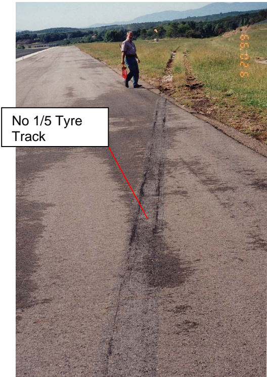
Figure 24.1 – Runway Edge Tracks
