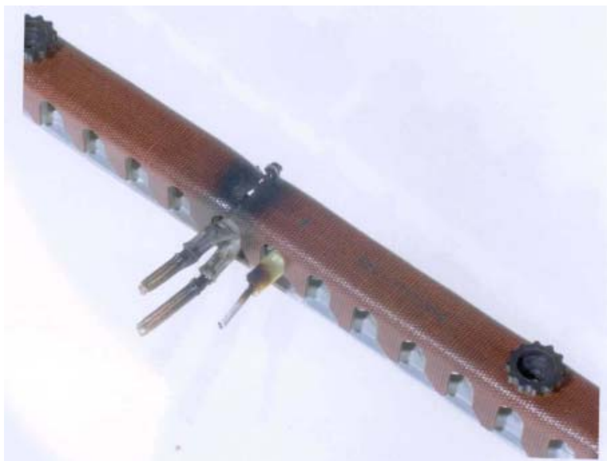
Fig. 2 Terminal Board with heat damage
